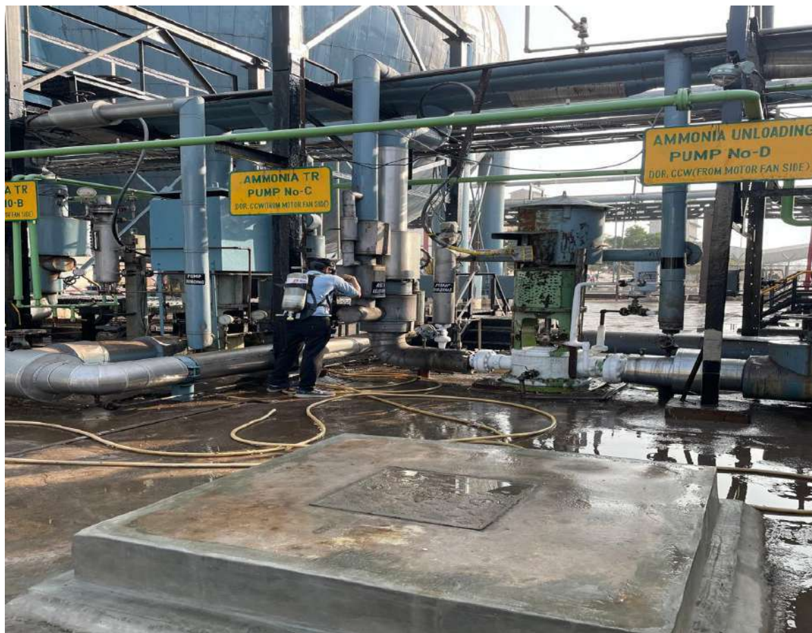
Area Operator Closing Isolation valve to isolate pump
