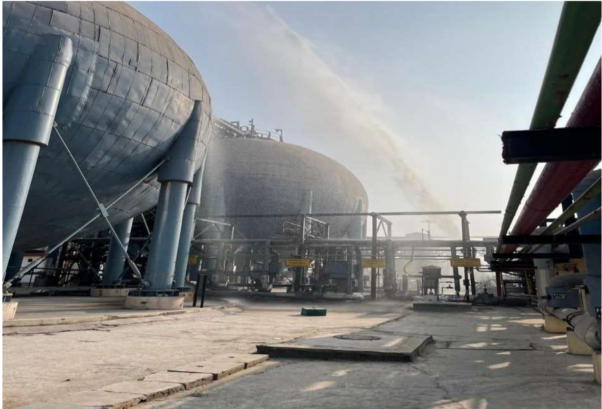
Water Monitor started at Horton Sphere.
