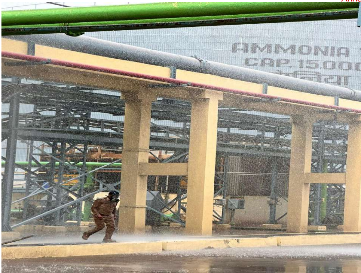
Fire Crew Diluting Ammonia Vapors with Water Spray
