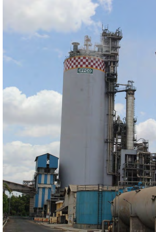
Urea Prill Tower with Vibro Priller
