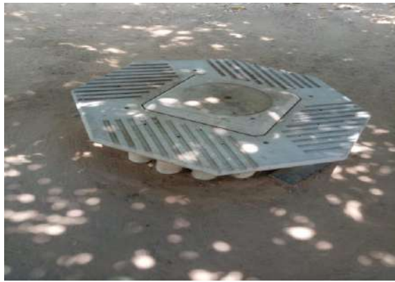
Module installed near Sr. GM Bungalow
