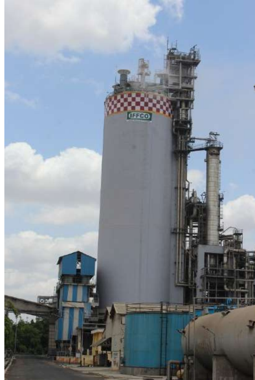
Urea Prill Tower with Vibro Priller
