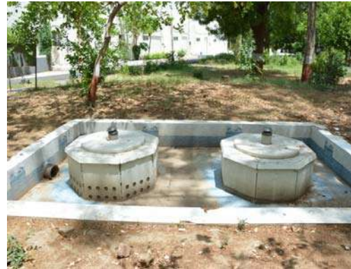
Rain Water Harvesting system (New) (25 m 3 /hr capacity)
