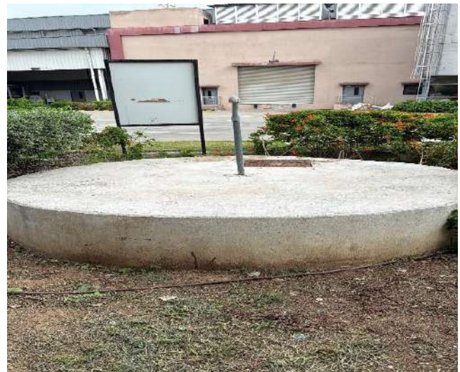
(Recharge well near Air washer)
