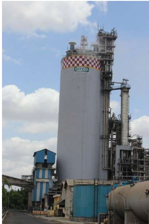
Urea Prill Tower with Vibro Priller
