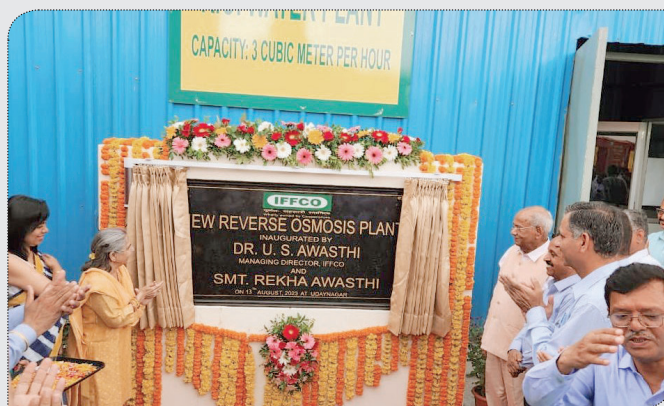
IFFCO Managing Director Dr Udai Shanker Awasthi inaugurated the new RO water treatment plant at Udayanagar Township during the IFFCO Kandla visit. This will help in providing better quality drinking water to all in the township.
